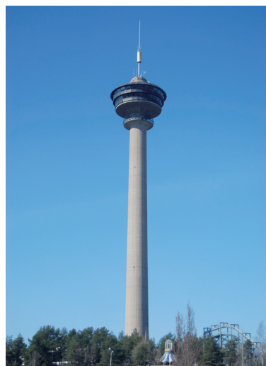
Fig. 3. Näsäinneula Observation Tower, one of the landmarks in Tampere.
