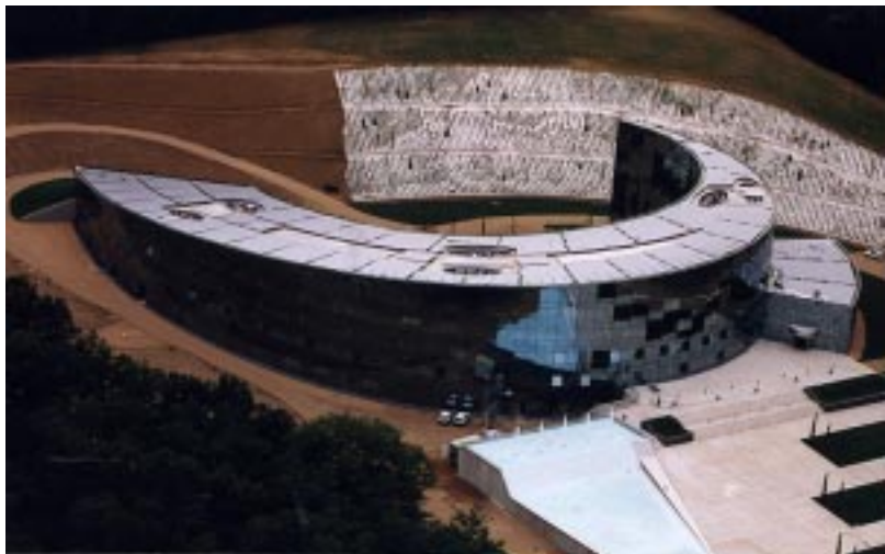
Fig. 1. The newly built head office of the Pierre Fabre company, in the green surroundings of Castres. The whole building is a sculpture inspired by the yang-yin symbol.
